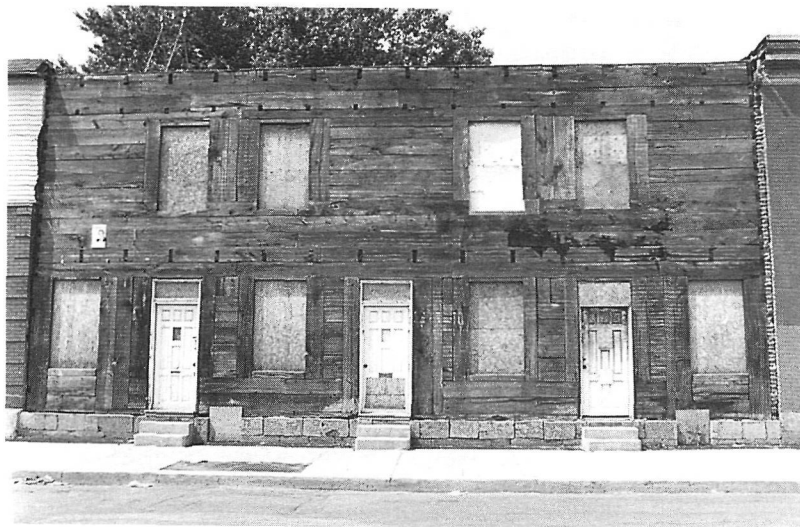
Working-class homes of the 1872 boom were still of plank construction “pièce sur pièce” as shown for a double-duplex on Liverpool street; the brick cladding has been removed, for replacement.
