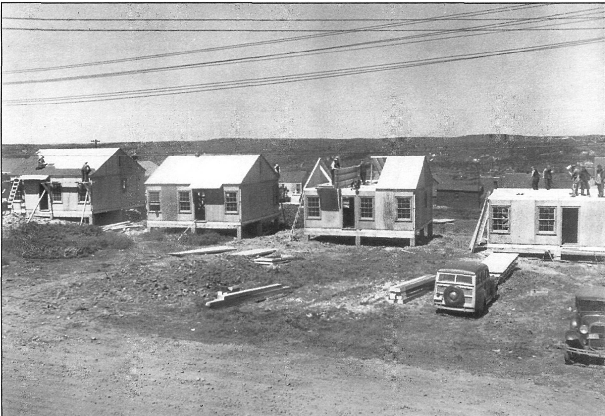
Figure 1: “Construction by the Wartime Housing Ltd. of prefabricated houses for munitions workers, Canada.” Cbicoutimi, March 1942. Note the stages of construction, from right to left, and the alternation of doorways and middle windows.
