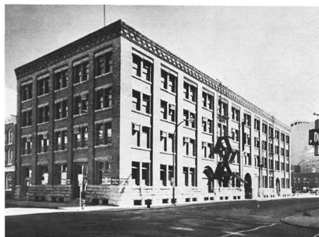
FIGURE 8. George D. Wood Warehouse in 1977
