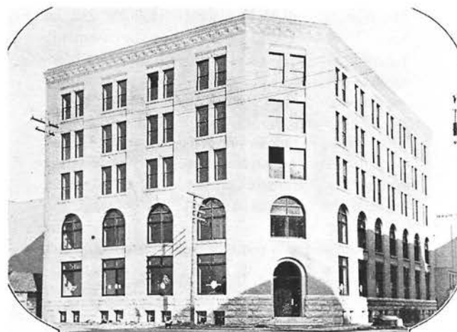
FIGURE 9. F.W. Stobart Warehouse. Architect: J.H. Cadham
