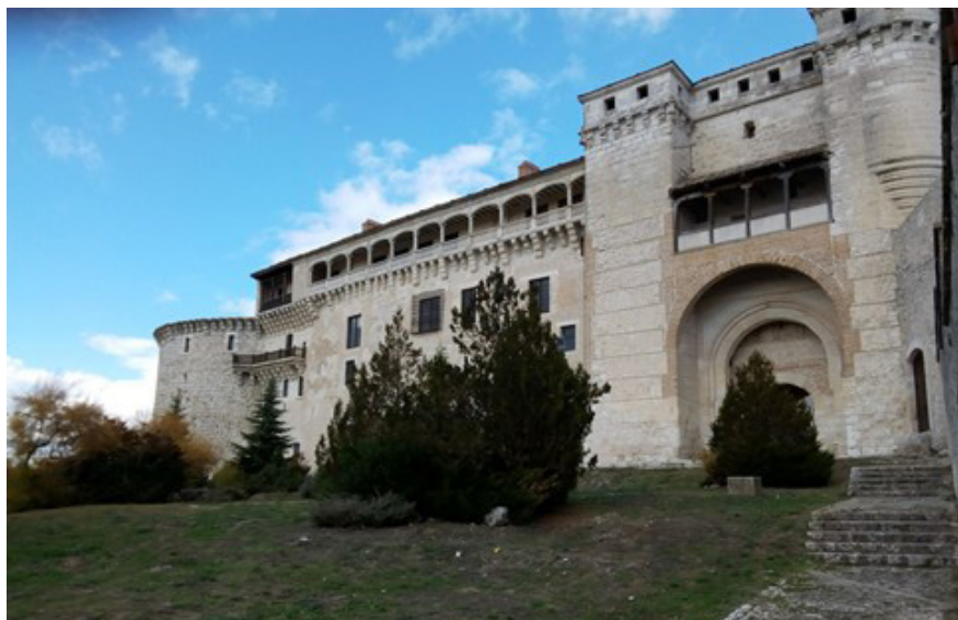
Figure 2. The gallery on the southern wall of the castle, towards the gardens. Castle of the dukes of Albuquerque, Cuéllar (Segovia).
