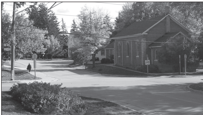
FIGURE 10. Looking southward along Second Line where it crosses Old Derry Road, in 2012. This might have been the intersection of two six-lane arterial roads. The 1863 Methodist Church stands on the southwest corner, with the 1871 village school (later, community hall) visible beyond. (Author photo)
