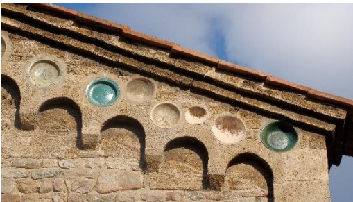
Figure 3 San Sisto, detail of bacini decoration on west façade. Photo by author.
