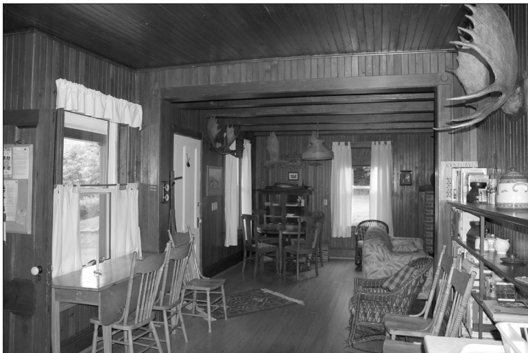
Fig. 35 Interior view of ca. 1930s alterations to the SE side of the double house. Note the widened passage between kitchen ell and dining room, darkly stained boards, boxed beams, and the edge of the fireplace mantel. Photo by author.
