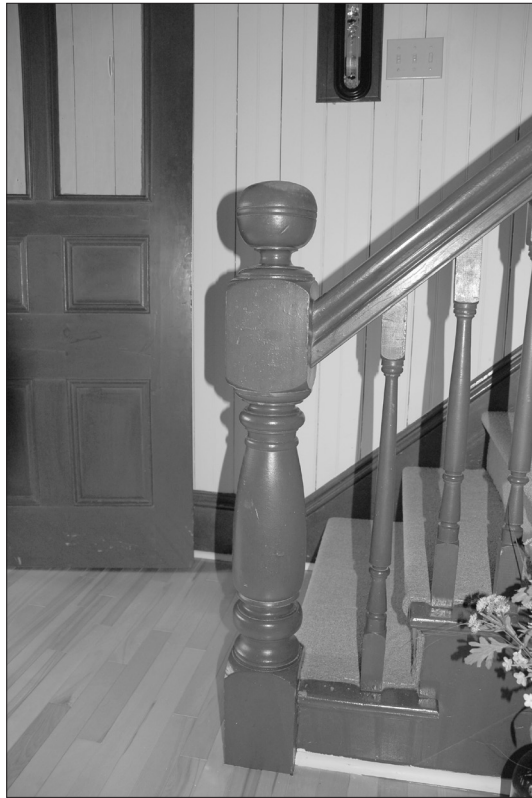
Figs. 28a (below left), b (below right) Stair newel post and balustrade, NW (right) side of house. (b) Stair newel post and balustrade, SE (left) side of house. Photos by author.
