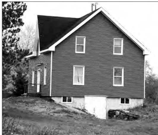
Fig. 9 The Fraser farmhouse, East River St. Mary's. Vinyl siding and windows, as well as a raised concrete basement are part of the recent renewal. Photo by author.
