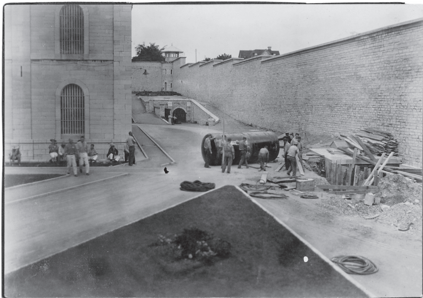
Kingston Penitentiary, 25 October 1933. The prisoners on the left are taking their break outside the south face of the prison hospital, while on the right an excavation team prepares to install a new oil drum.
