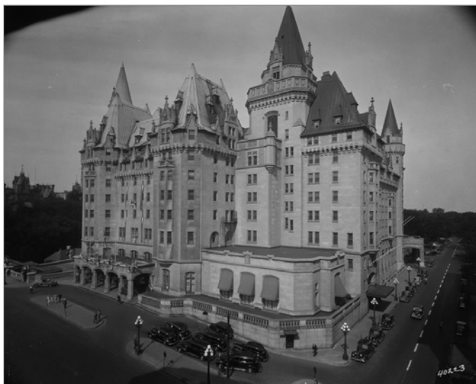
FIG. 6. THE 1929 ADDITION TO CHÂTEAU LAURIER, PHOTO TAKEN 1937. | CANADIAN NATIONAL RAILWAY COMPANY, LIBRARY AND ARCHIVES CANADA, R231-2009-6-E, BOX NUMBER: INT 014, RV4 52-1.
