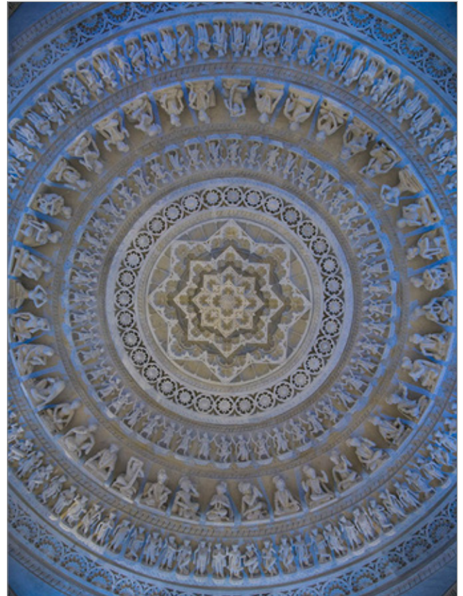
FIG. 13. CEILING OF CORBEL CONSTRUCTION USED TO TRANSITION FROM A SQUARE TO A CIRCLE. | BAPS TORONTO. COPYRIGHT HELD BY BAPS SWAMINARAYAN SANSTHA.
