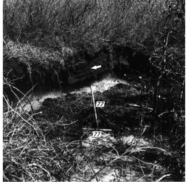
FIGURE 54. BM 77 (Fig. 53b) broken by the growth of 0.75 m of intrusive ice in the winter of 1975/76 as a result of renewed normal faulting along "dilation crack x" (Fig. 40). The arrow points to the location where the top of BM 77 was broken off. The broken top is labelled "77" and is horizontal at the bottom of BM 77. The water source was along the fault as shown in Figure 55.
