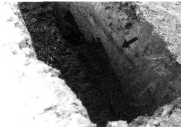
FIGURE 4. View of sub-surface stratigraphy in a back-hoe trench showing a horizontally bedded, organic-rich layer in Unit 4 (photograph from Veillette and Nixon, 1984).
