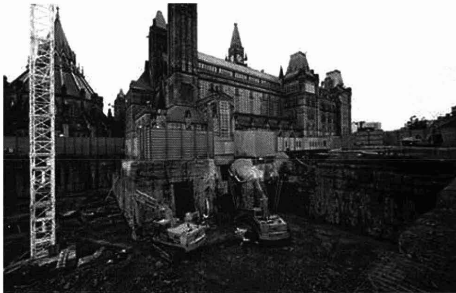
Figure 17 Excavation for the Centre Block Underground Services space (CBUS) involved the removal of about 30,000 m 3 of rock during a 3-month period in 1997. PWGSC 1997.
