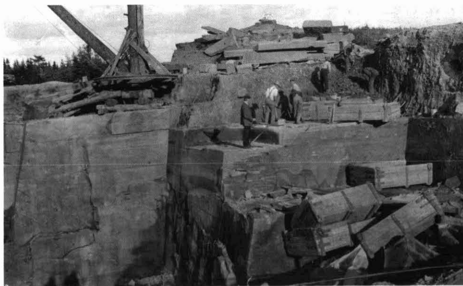
Figure 7 Quarrying sandstone at the Wallace Quarry, Nova Scotia. This stone was used in part as a replacement for Ohio Sandstone on the reconstructed Centre Block and Peace Tower. J. Keele, 1909, Geological Survey of Canada.
