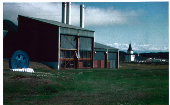
Figure 8 (at left) Photo/diagram schematic through one of the Vestmannaeyjar heating units. Figure 9 (above) The geothermal water distribution plant in central Vestmannaeyjar.
