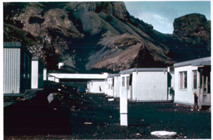
Figure 7 Temporary housing in west Vestmannaeyjar, August 1974.
