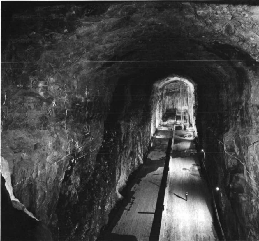
Figure 1. Typical Swedish rock cavern for storage of petroleum products. (Photo courtesy of Skanska Cementgjuriet.)
