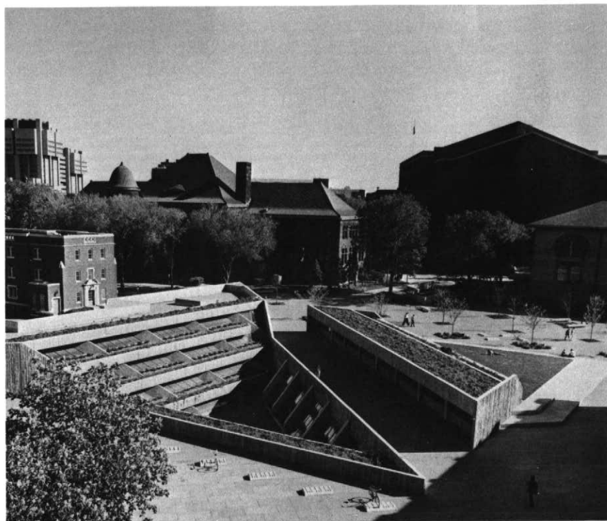
Figure 3. Underground three-storey Bookstore and Office Building on the main campus of the University of Minnesota, Minneapolis (opened 1977). (Photo courtesy of the University of Minnesota.)
