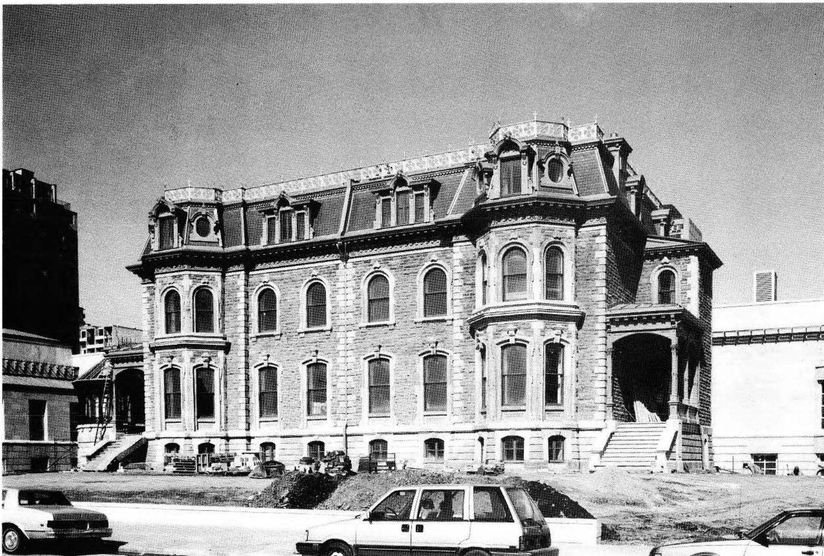
FIGURE 222. Alain Laforest, Canada, Montréal 1952- , Canadian Centre for Architecture, Montréal: View of South Elevation Showing the Shaughnessy House, Looking Northwest , Peter Rose Architect, gelatin silver print, 20 April 1989, 14.6 × 22.6 cm. 20/04/89-01-A1-25, Collection Centre Canadian d'Architecture/Canadian Centre for Architecture, Montréal.
