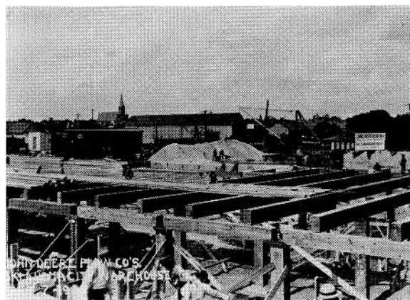
FIGURE 6. Basic Framing, John Deere Plow Co. Warehouse, July 7, 1906.
