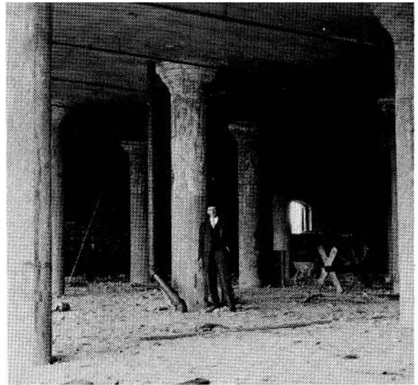
FIGURE 18. Construction Photographs of Spokane Warehouse for John Deere Plow Co.
