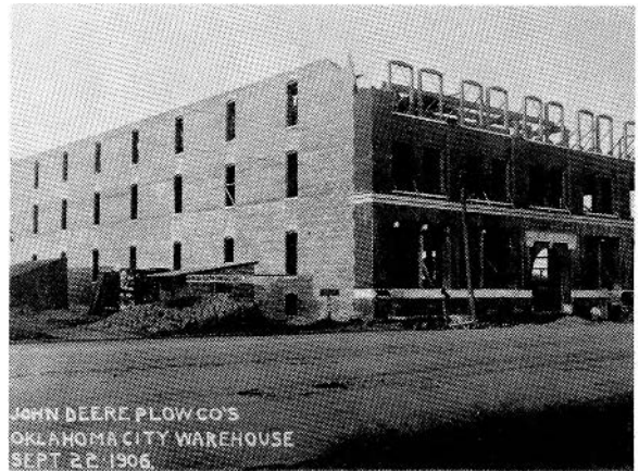
FIGURE 7. Deere Warehouse, Oklahoma City at completion of first two storeys, Sept. 22, 1906.
