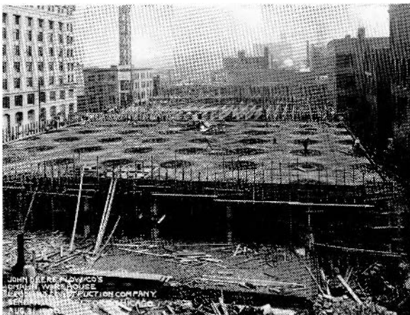
FIGURE 10. Omaha Warehouse under construction, Aug. 31, 1908.
