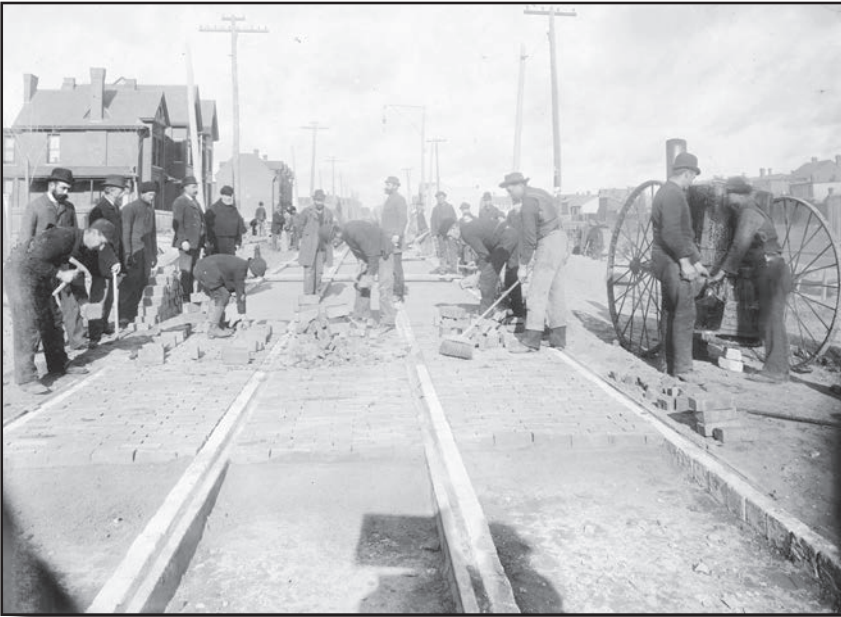
Not Craiggellachie but part of a civic dream, streetcar tracks along Bathurst Street. City of Toronto Archives Fonds 200 Former City of Toronto fonds. -1834-1997, Series 376 City Engineer's Dept. photographs. - 1891-1911, File 1, Item 18
