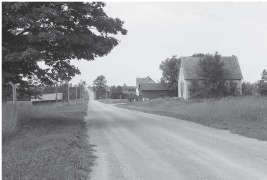
FIGURE 2. Williscroft Baptist church (1907) stands abandoned, square to the squared-off Ontario landscape. Lot 9, looking west along the 12th Concession Line, Elderslie Township, Bruce County, 1983.
