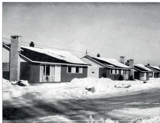
FIG. 9. THE AWARD-WINNING BRAD HOUSES IN 1959 (W.G. COOK, ARCHITECT). SLAB-ON-GRADE CONSTRUCTION WAS NOT POPULAR WITH OROMOCTO'S CIVILIAN BUYERS, WHO APPRECIATED A BASEMENT AND LOWER HEATING COSTS IN COLD NEW BRUNSWICK WINTERS. | "CANADIAN HOUSING DESIGN AWARDS - HOUSE GROUPING" HABITAT, VOL. 11, NO. 4, JULY 1959, P. 21.
