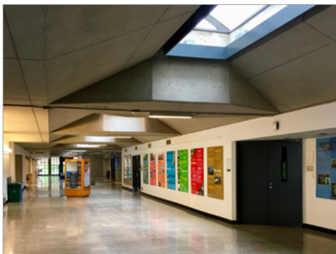
FIG. 13. "THE STUDENT STREET," LOOKING SOUTH, MACKINTOSH-CORRY HALL (R.J. THOM ARCHITECTS, 1972-1974), QUEEN'S UNIVERSITY, KINGSTON. | JAMES ASHBY, 2019.
