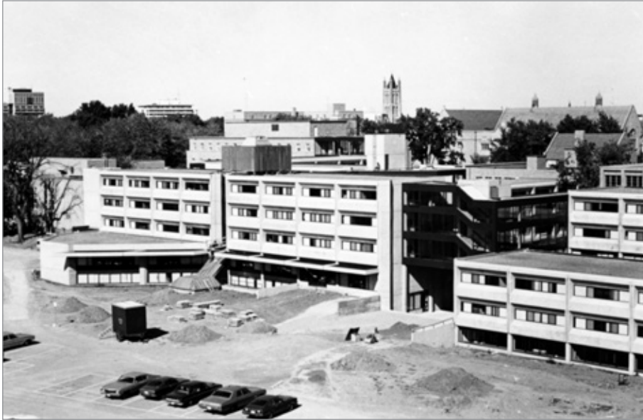
FIG. 7. VIEW OF ARTS AND SOCIAL SCIENCES COMPLEX (R.J. THOM ARCHITECTS, 1972-1974, TODAY MCINTOSH-CORRY HALL) LOOKING EAST, QUEEN'S UNIVERSITY, KINGSTON. | UNKNOWN PHOTOGRAPHER, C. 1974, QUEEN'S UNIVERSITY ARCHIVES, V28-B-MACKIN-4, QUEEN'S PICTURE COLLECTION, BUILDINGS, MACKINTOSH-CORRY HALL.
