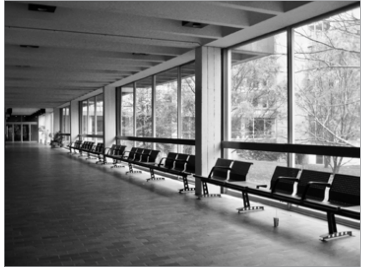
FIG. 9. GROUND FLOOR CORRIDOR WITH COURT BEYOND, ARTS BUILDING (TODAY MACKINNON BUILDING) (SERT JACKSON AND ASSOCIATES INC. WITH HANCOCK LITTLE CALVERT ASSOCIATES, 1967), UNIVERSITY OF GUELPH, GUELPH. | JAMES ASHBY, 2012.
