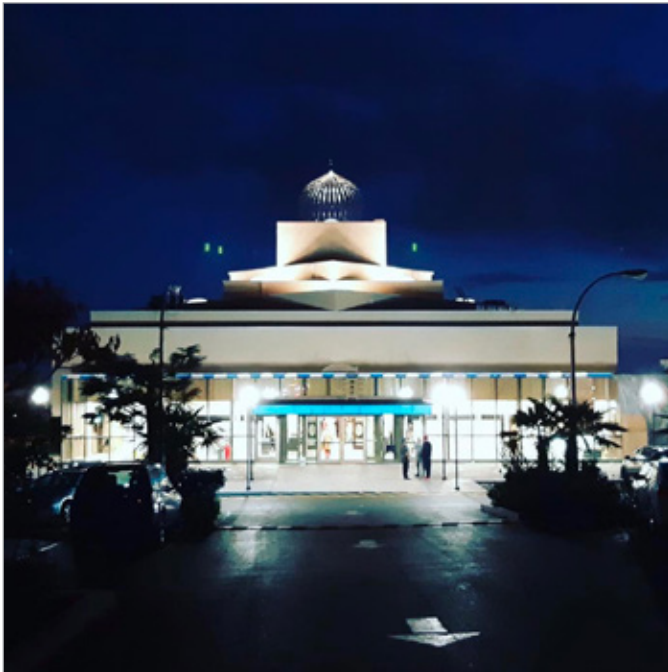
FIG. 26. AT NIGHT, THE NORTH ELEVATION OF THE KHALSA DIWAN SOCIETY VANCOUVER GURDWARA, 8000 ROSS STREET [KHALSA DIWAN ROAD], VANCOUVER, SHOWING THE STEEL AND GLASS PAVILION NOW FRAMING THE MAIN ENTRANCE: [HTTPS://WWW.FACEBOOK.COM/KDSROSS/PHOTOS/4854923237868748]. | THE KHALSA DIWAN SOCIETY VANCOUVER.
