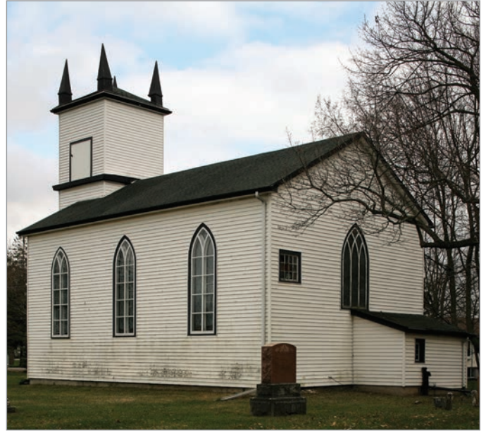
FIG. 14. PORT ROBINSON, ST. GEORGE'S ANGLICAN CHURCH, EXTERIOR FROM SE. | MALCOLM THURLBY.
