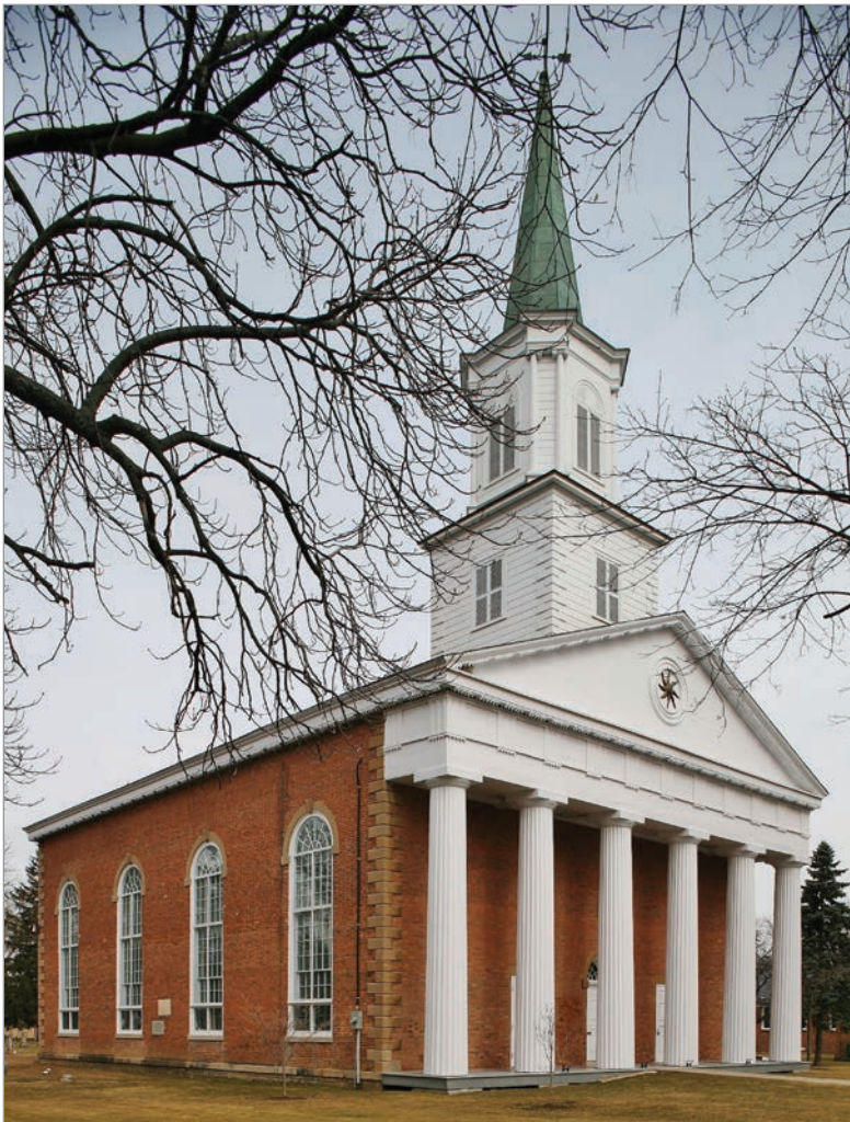
FIG. 1. NIAGARA-ON-THE-LAKE, ST. ANDREW'S PRESBYTERIAN CHURCH, 1831, EXTERIOR FROM SE. | MALCOLM THURLBY.
