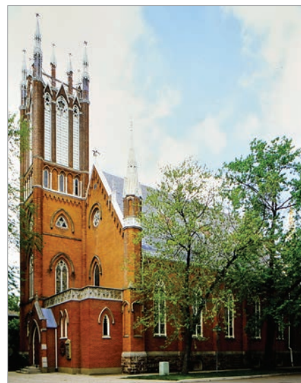
FIG. 37. ST. CATHARINES, WELLAND AVENUE METHODIST (UNITED) CHURCH, 1878, EXTERIOR. | MALCOLM THURLBY.
