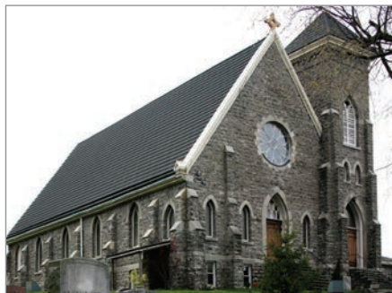
FIG. 36. FORT ERIE, ST. PAUL'S ANGLICAN, 1878, EXTERIOR. | MALCOLM THURLBY.
