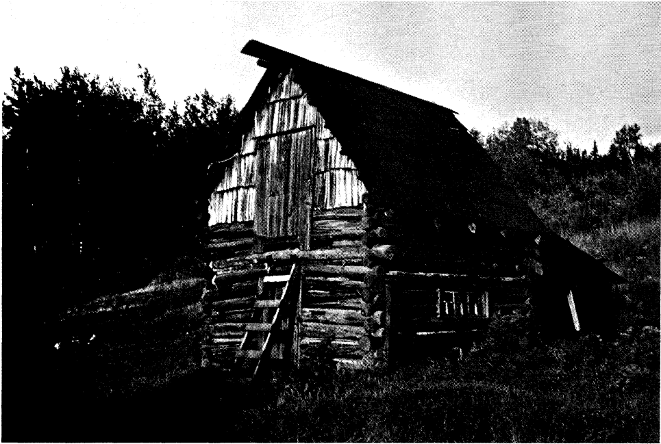
Photo 6 Barn with extended ridge-pole at La Macaza, Joly.
