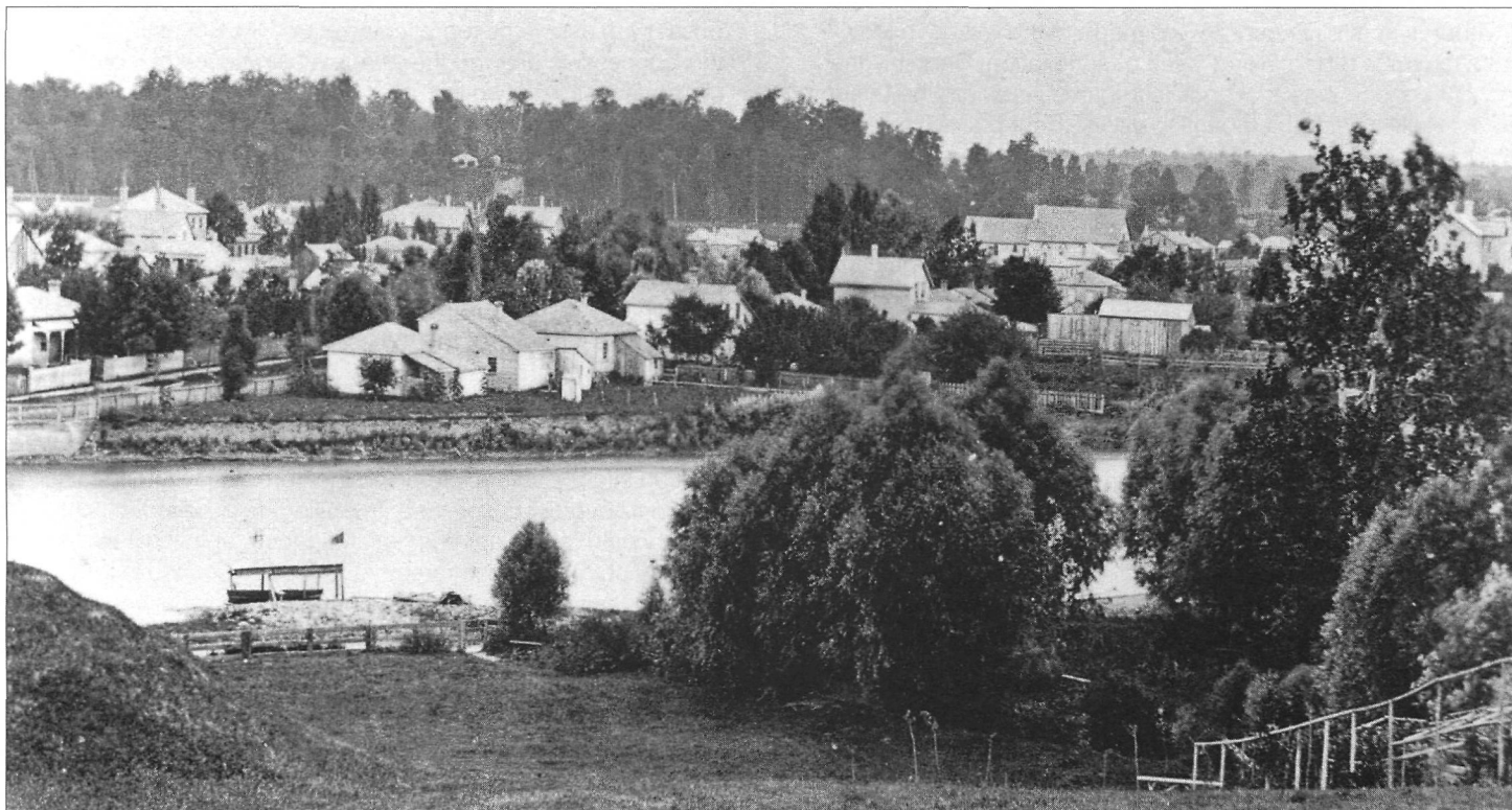
Figure 2: A view of London West (circa 1880) looking west. Running from the far left is Ann Street. Top right is the two-story Ann Street school, to the left of which the Methodist Church is visible. Note the striking height difference between the east and west banks of the Thames. Courtesy of the J. J. Talman Regional Collection, the D. B. Weldon Library, the University of Western Ontario
