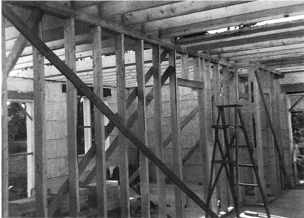
Figure 12: By late Sunday afternoon the first floor was framed, Summer 1949.
