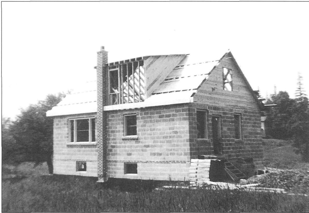
Figure 13: The house as it approached completion in late summer 1949. Owner-builders like the Halls favoured concrete blocks since they were comparatively cheap and easy to lay.
