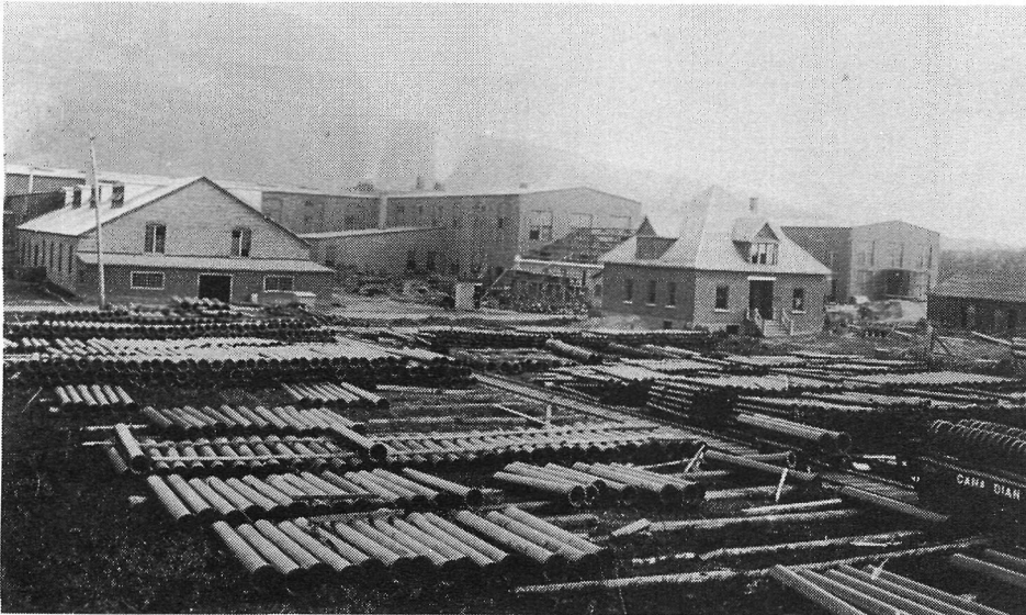
The Canadian Iron and Foundry Co. (later part of the Canada Iron Corporation) was bonused in 1906 and in operation by 1907 producing mainly rail car wheels and cast iron pipes for the western Canadian market. (Thunder Bay Historical Museum Society, 977.113.216)
