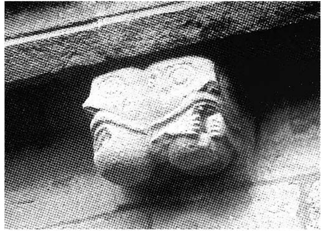
Figure 7. Corbel no. 8 of the south nave (tongue-protruder). St. Nicholas, Studland (Photo: Malcolm Thurlby).
