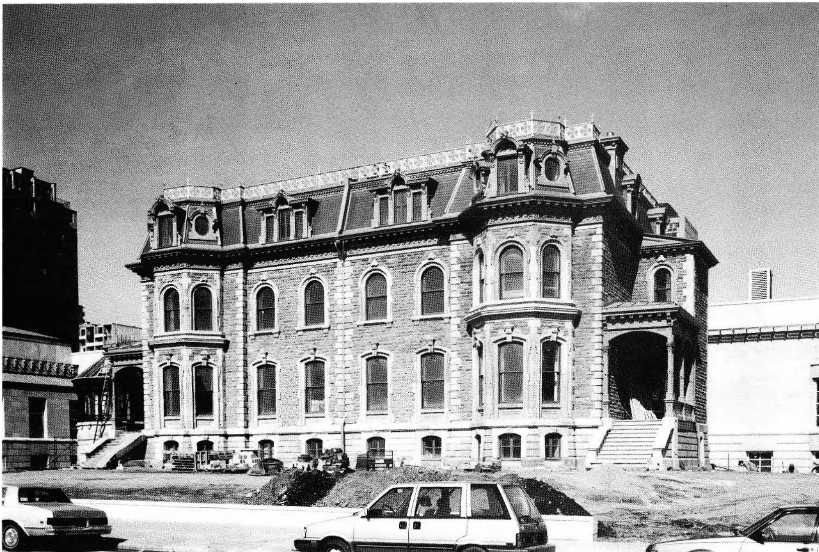
FIGURE 222. Alain Laforest, Canada, Montréal 1952- , Canadian Centre for Architecture, Montréal: View of South Elevation Showing the Shaughnessy House, Looking Northwest , Peter Rose Architect, gelatin silver print, 20 April 1989, 14.6 × 22.6 cm. 20/04/89-01-A1-25, Collection Centre Canadian d'Architecture/Canadian Centre for Architecture, Montréal.
