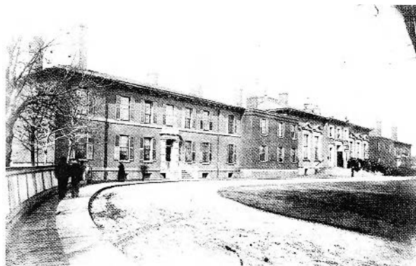
FIGURE 1. Third Parliament Buildings, Toronto. Exterior view, 1884. Metropolitan Toronto Library (Photo: Metropolitan Toronto Library).
