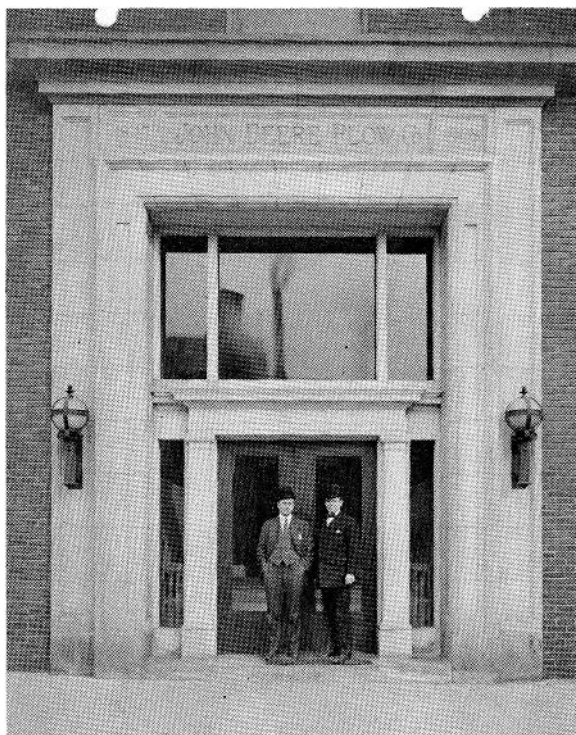
FIGURE 13. Entryway, Deere warehouse, Omaha.
