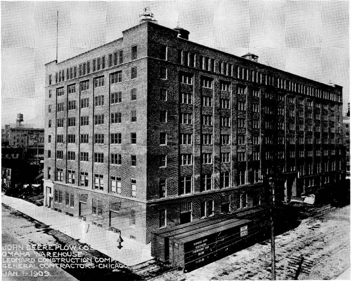
FIGURE 9. Omaha Warehouse for John Deere Plow Co., Omaha, Jan. 1, 1909. Oscar A. Eckerman, Architect.
