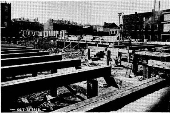
FIGURE 2. Construction Photograph, St. Louis Warehouses.
