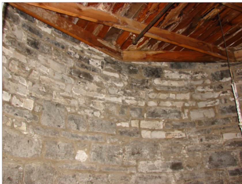
FIG. 18. ST. GEORGE'S CHURCH, 1839-1841; DETAIL OF THE INTERIOR OF THE TAPERED CIRCULAR WALL WHERE IT MEETS THE FLOOR OF THE BELFRY. | PHOTO: PAUL CHRISTIANSON, NOVEMBER 2020.
