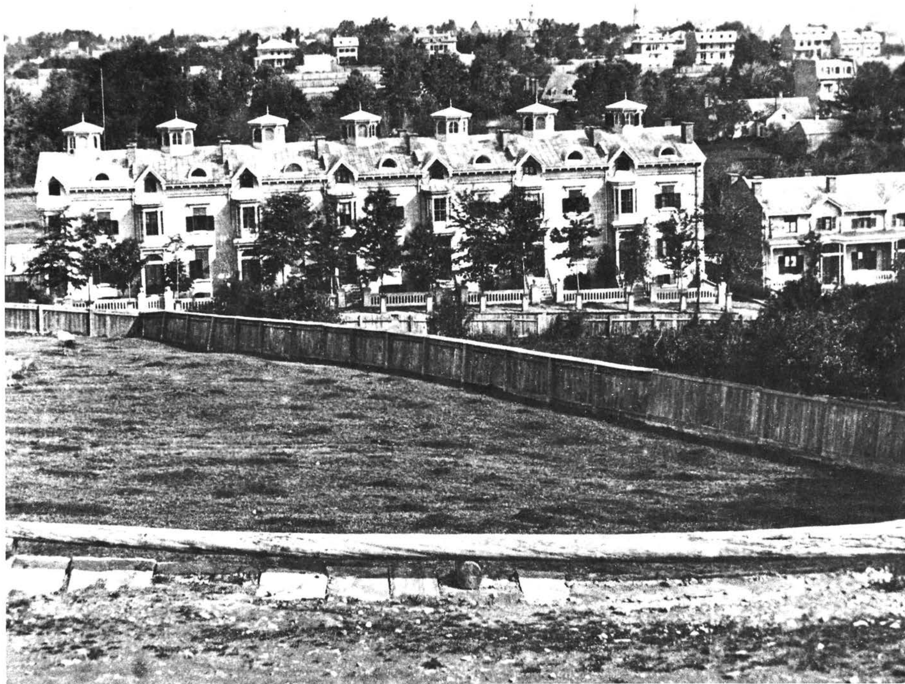
McGill College Avenue looking north from St. Catherine Street at "Mount Royal Terrace," built in 1858-59, and "St. Sophie Place," built in 1858. Photo: Walker, c.1865. (Source: McCord Museum, Montreal)
