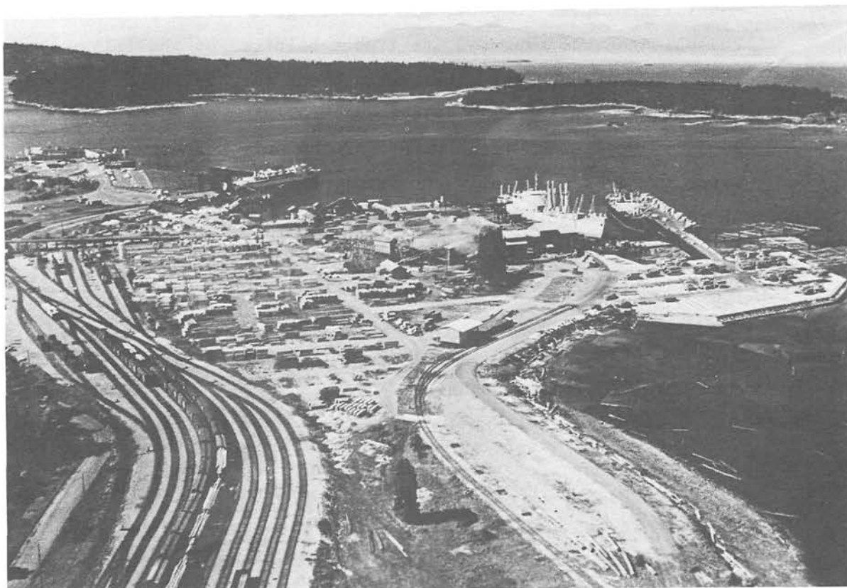
Photograph #5: Deepsea Lumber assembly wharf and rail and motor vehicle ferry terminuses are the key to Nanaimo's post war expansion as a trans-shipment point and distribution centre. Most of the complex was built on mine waste fill, much of it from No. 1 mine which was located to the left of the curve in the tracks. Other coal mines were on Newcastle and Protection Islands across the harbour. (Victoria Press Limited photograph).
