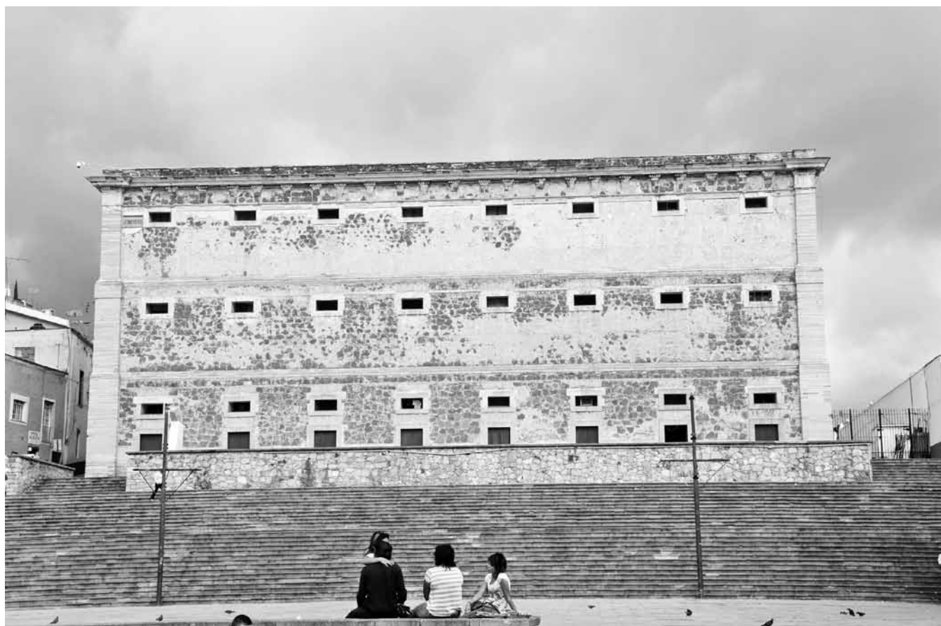
Figure 8. Granary of Granaditas, Guanajuato. West façade (Photo: author).
