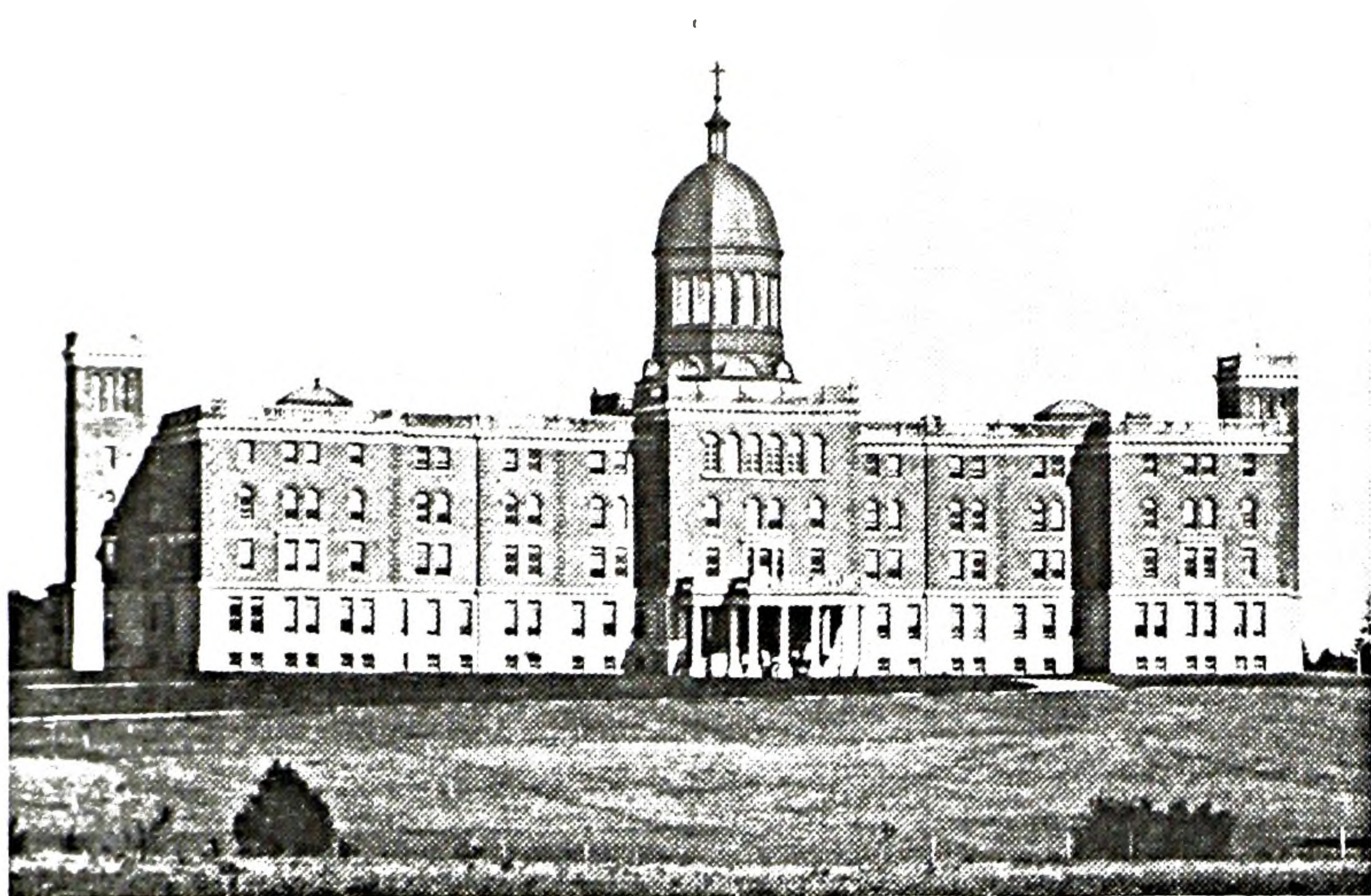
FIGURE 21. St. Augustine's Seminary. General view from the west, after Construction , VIII (December 1915), p. 486 (Photo: Metro Toronto Library Board).
