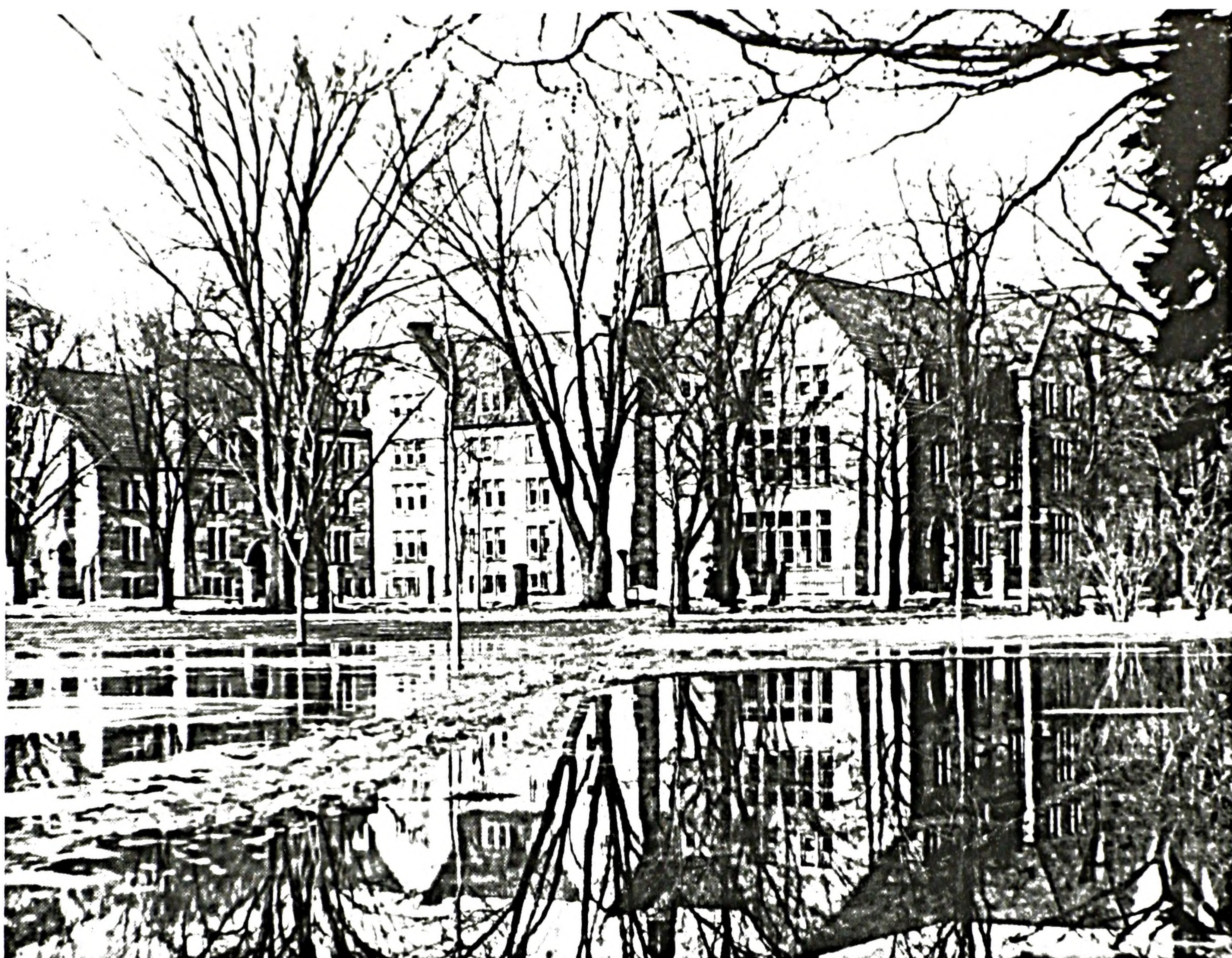
FIGURE 34. A.W. Holmes, 'Queen's Park Buildings', St. Michael's College, Toronto. Main front as in 1942. Archives of St. Michael's College, photo 1942-12 (Photo: author).
