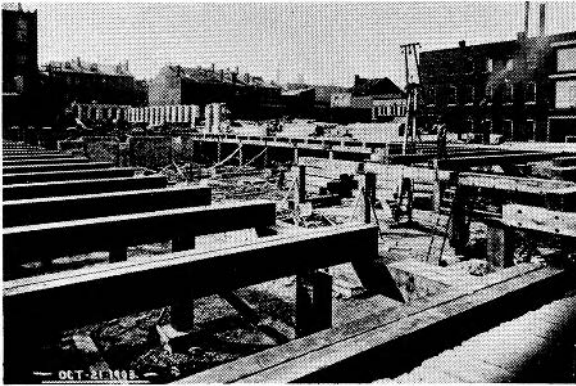
FIGURE 2. Construction Photograph, St. Louis Warehouses.
