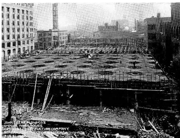
FIGURE 10. Omaha Warehouse under construction, Aug. 31, 1908.
