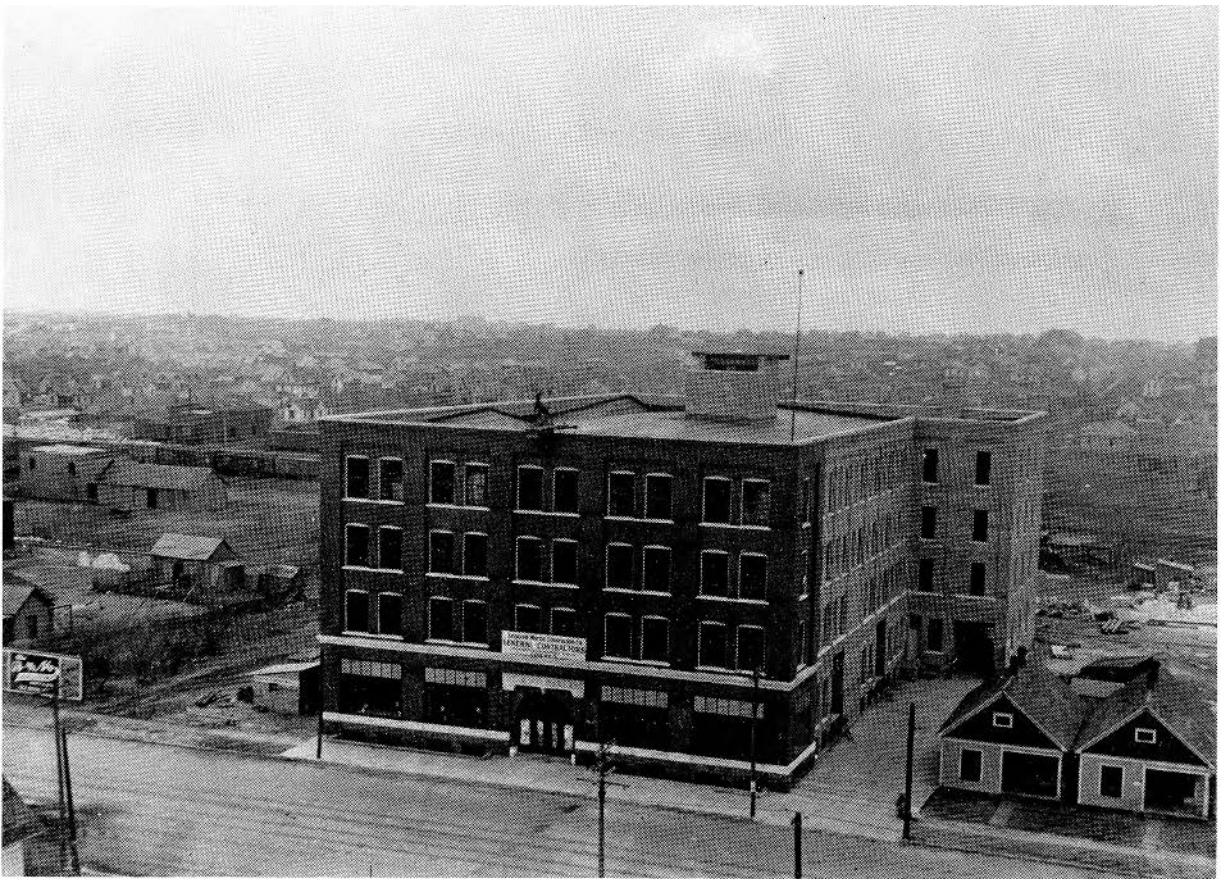
FIGURE 8. Completed Warehouse for John Deere Plow Co., Oklahoma City, Dec. 5, 1906.
