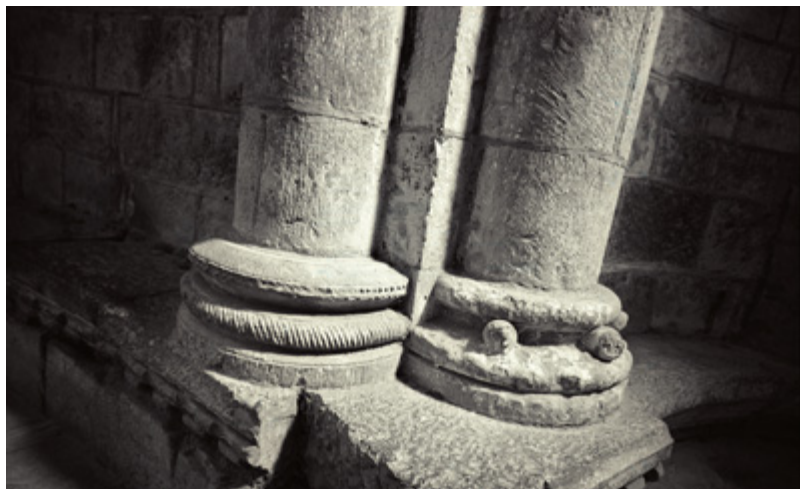
Photo 2: Columns in Nave
