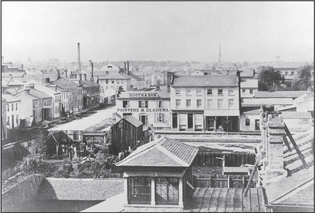
Booth & Son: north-east corner of Adelaide and Victoria streets in 1856. This is the street that the Mansion House Livery Stable was on, next to Booth & Son. Courtesy of City of Toronto Archives, Fonds 1498, Item 6.
