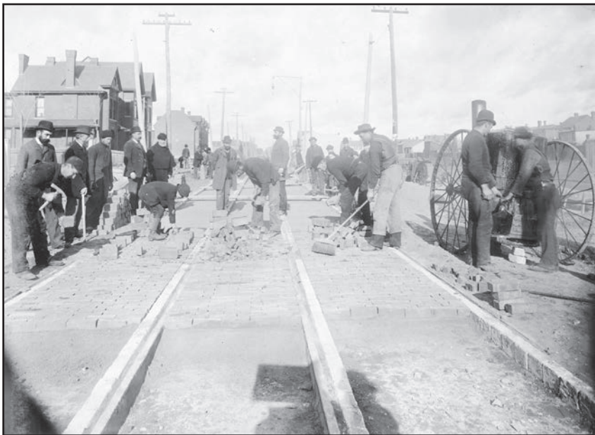
Not Craiggellachie but part of a civic dream, streetcar tracks along Bathurst Street. City of Toronto Archives Fonds 200 Former City of Toronto fonds. -1834-1997, Series 376 City Engineer's Dept. photographs. - 1891-1911, File 1, Item 18
