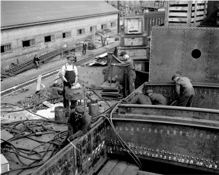
Men at work on a 10,000-ton dry cargo ship in a Montreal shipyard. Note the burner at left operating an oxy-acetylene torch. Behind him standing on deck is a heater with his portable furnace for heating rivets. At the right a group of workers include a riveter and a holder on.
