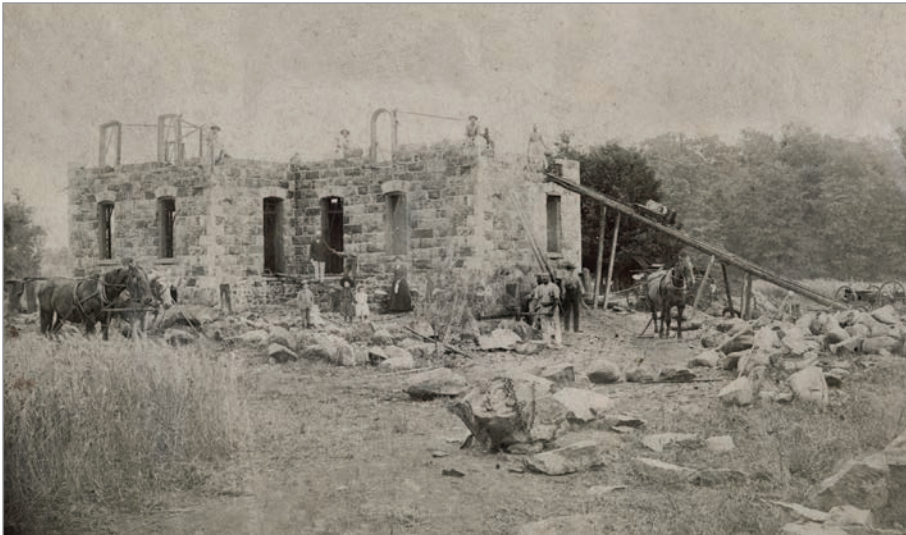
FIG. 20. ALEXANDER SUTHERLAND HOUSE, CONSTRUCTION SITE, 1891, ROAD 74, NO. 4358, GOLSPIE, OXFORD COUNTY. | SPECIAL THANKS TO KEN JUDGE.
