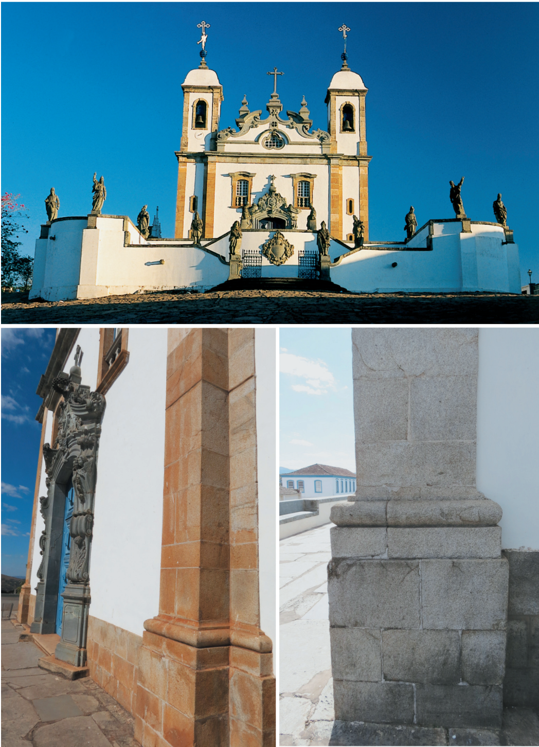
Figure 7. Example of patina formation (oxidation), deposition of particles, and biological colonization on the surface of granite blocks with whitish-grey original colour, on the frontispiece of the Congonhas Sanctuary of Bom Jesus church. The current brownish colour (patina) results from the position of these (outer) blocks facing the action of wind currents and variations in moisture content. In areas unaffected by such currents, the granite retains its original whitish-grey colour, although it is susceptible to intense biological colonization.
