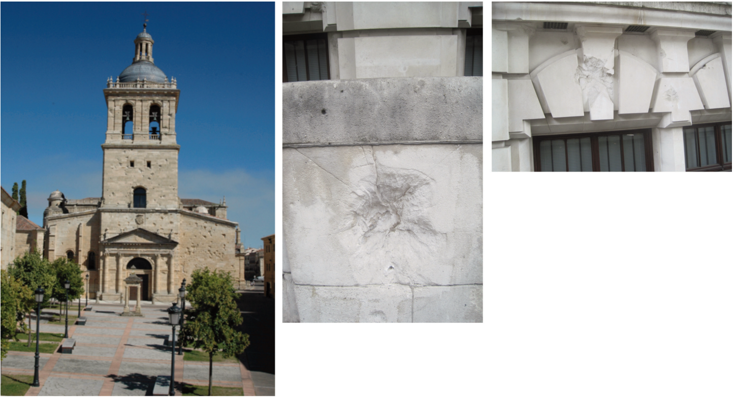
Figure 1. Examples of war damage: a) Cathedral in Ciudad Rodrigo (Salamanca, Spain) showing cannon ball impacts from the siege during the Peninsular War between French and Anglo-Portuguese and Spanish forces in the early 19 th century. b) and c) parts of the façade of the Victoria and Albert Museum in London showing damage to the Portland Stone from casing fragments when bombs were dropped nearby. The damage was deliberately left unaltered when the façade was cleaned and repaired in 1985.
