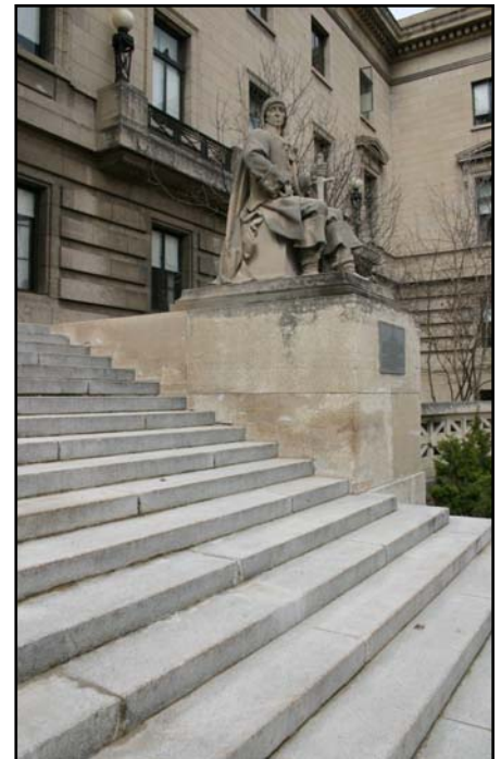
Figure 3. Statuary of Bedford limestone sits on a pedestal of Tyndall Stone at the east entranceway. The stairs are made of Butler granite.
