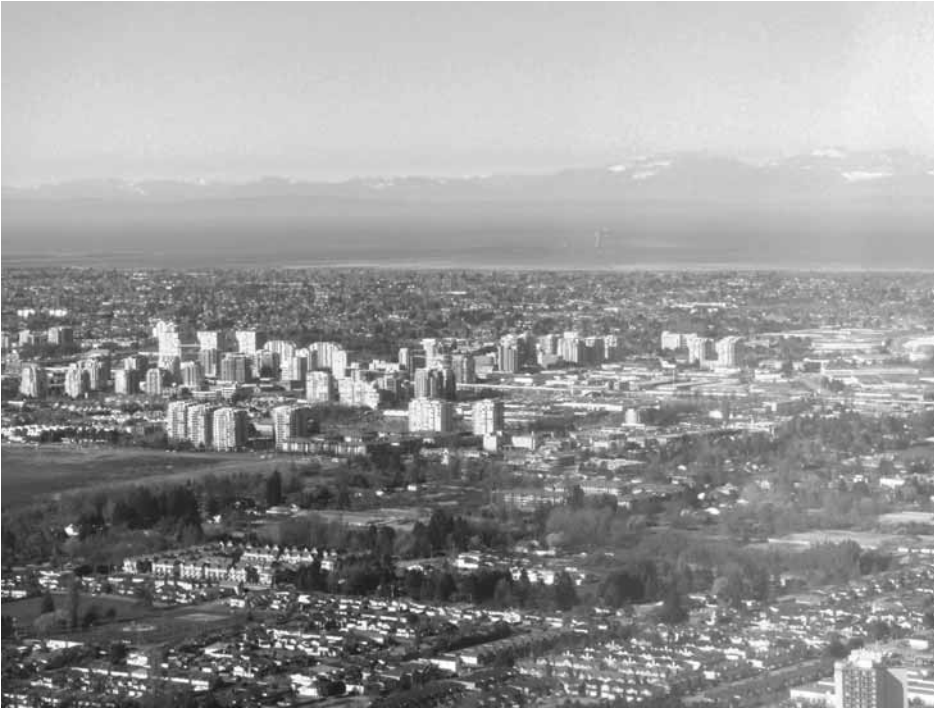
Figure 11. Richmond, British Columbia. This rapidly growing city is less than 2 m above mean sea level and is protected from flooding by sea and river dikes. Photo by J.J. Clague.
