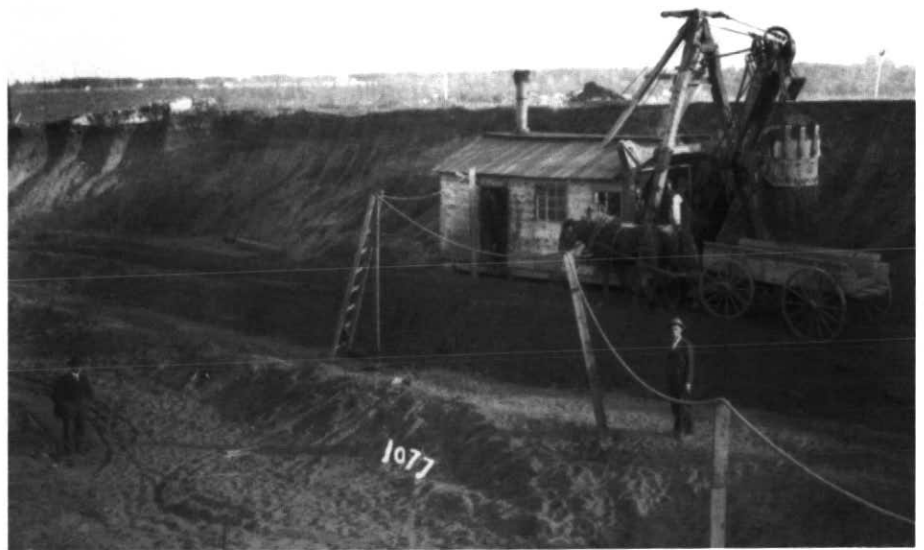
Figure 2 Steam-powered shovel excavating for the foundations of the Legislature (Provincial Archives of Alberta, B3354).
