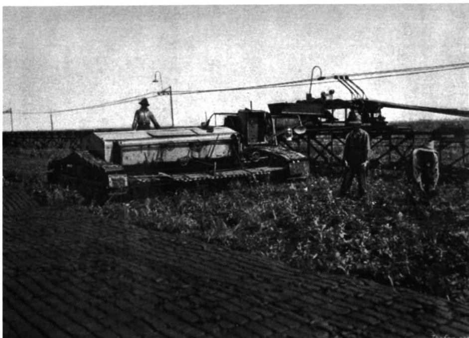
Figure 2 Spreading machine laying out peat to dry in the early 1920s at Alfred, Ontario (from Anonymous, 1928).
