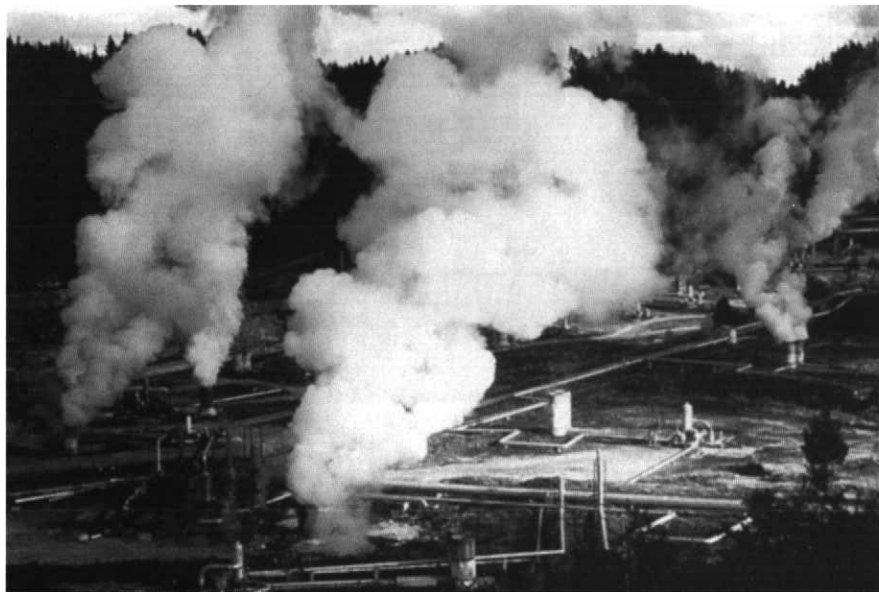
Figure 3 The well field at Wairakei, New Zealand, where wells have been drilled into a hot-water reservoir. The two-phase mixture is separated into its components in the separators, the small cylindrical objects. The large cylinders are noise mufflers for waste discharge.
